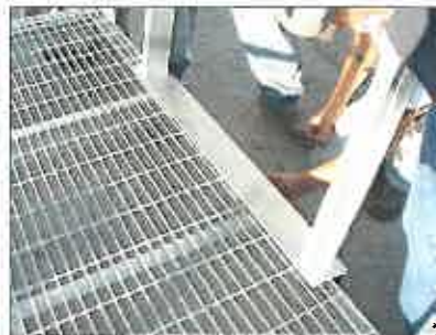
H-FRAME WILL REST RIGHT ABOVE WALK SURFACE
