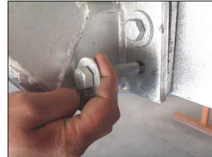
BOLT WITH \frac{1}{2} X2 \frac{1}{2} BOLTS AND TIGHTEN ALL CONNECTIONS WITH SOCKET AND WRENCH
