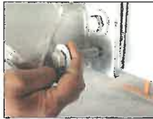
BOLT WITH \frac{1}{2} "X2 \frac{1}{4} " BOLTS AND TIGHTEN ALL CONNECTIONS WITH SOCKET AND WRENCH
