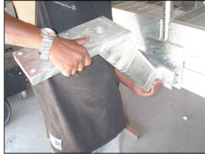
ALIGN HOLES IN GOOSENECK AND BASE
