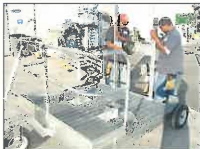
ALIGN H-FRAME INTO POSITION
