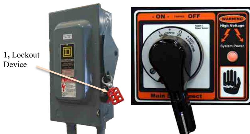
Figure 4-2, Typical Lockout Tag
